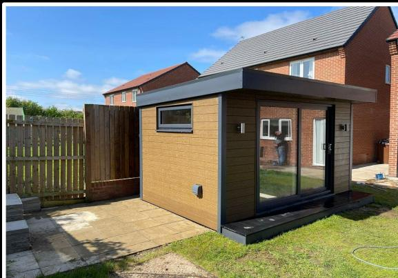
The 100mm structural timber walls and 120mm Tanelith E Treated floor sections are insulated with 75mm Knauf RS45 thermal acoustic insulation for superior warmth and soundproofing. Our garden pod roofs feature a highly insulated trapezoidal roof panel system, with a 120mm panel containing PIR rigid thermal insulation for maximum energy efficiency.
