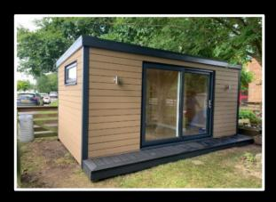
The 100mm structural timber walls and 120mm Tanelith E Treated floor sections are insulated with 75mm Knauf RS45 thermal acoustic insulation for superior warmth and soundproofing. Our garden pod roofs feature a highly insulated trapezoidal roof panel system, with a 120mm panel containing PIR rigid thermal insulation for maximum energy efficiency.
